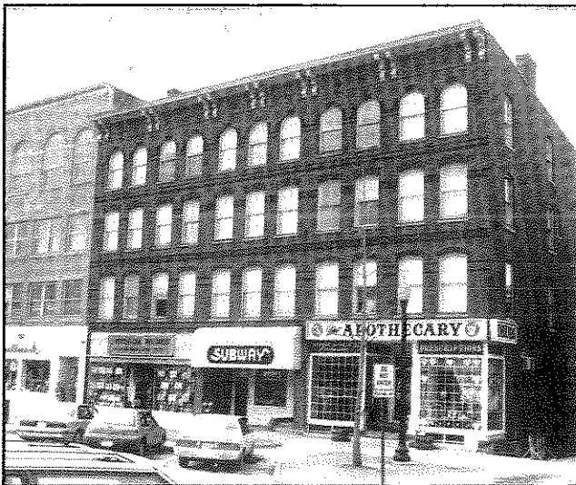
The Latchis building in Keene, New Hampshire, now owned by a bank as a result of foreclosure, is expected to provide affordable housing through Cheshire Housing Trust.
