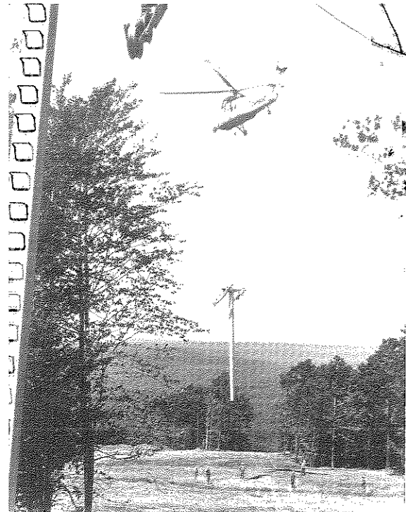
Left, placing lift towers by helicopter, 1972. Above, skiers disembarking from the dual double chairlift.
