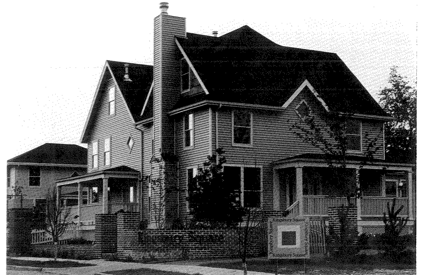
New homes in Kingsbury Square are part of the 106-acre De Baliviere Place redevelopment in central St. Louis.
