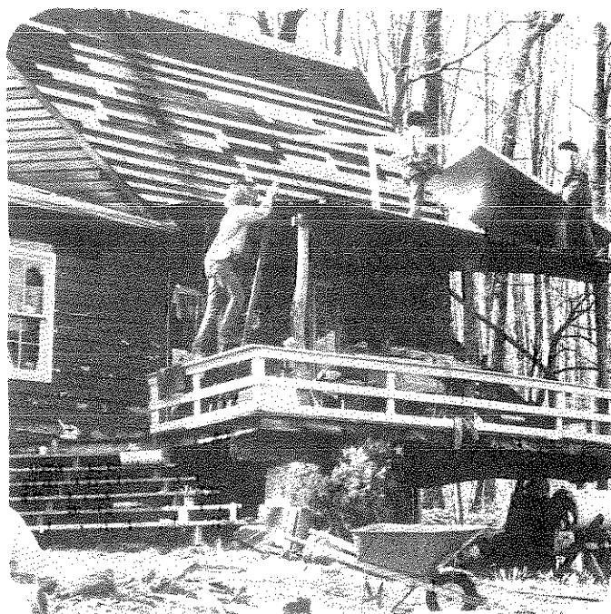
Raising of solar collector on roof of Hill House.
